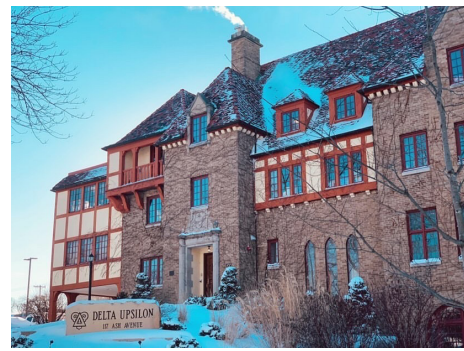
Full Facility at 117 Ash for 7 straight years
